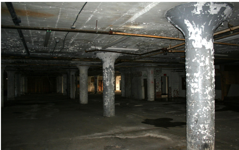
3. Concrete construction with mushroom columns.
