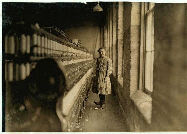
1. Typical slow burn construction interior in 1909.
